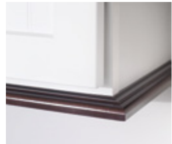
Under cabinet molding.
